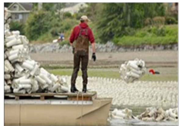
Figure 4: New Geoduck Installation, Eld Inlet, South Puget Sound (2013)
