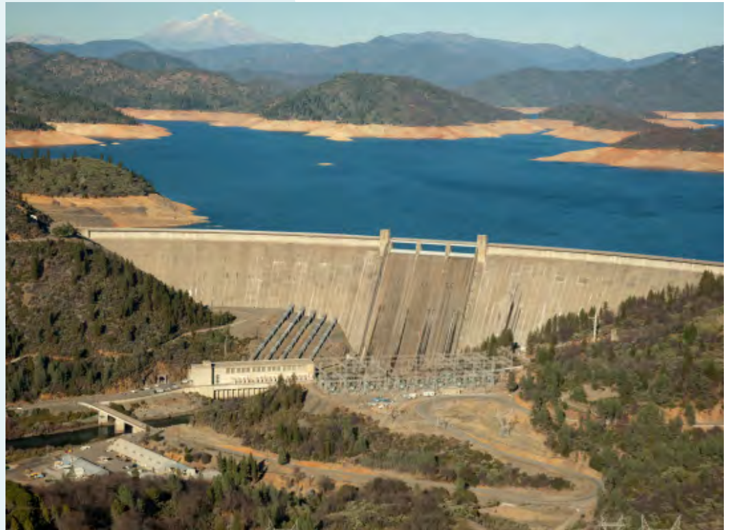
Upstream dams and diversions capture the majority of runoff in the Bay's watershed. Photo Credit: California Department of Water Resources
