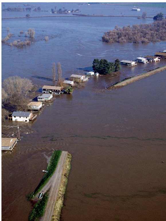
Delta levees are prone to failure, increasing risks to State water supplies.
