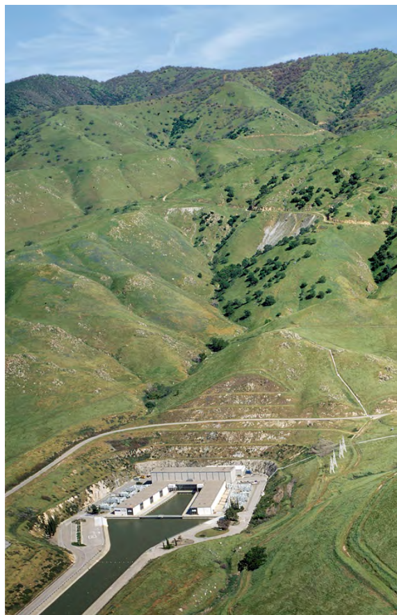
A. D. Edmonston Pumping Plant.
