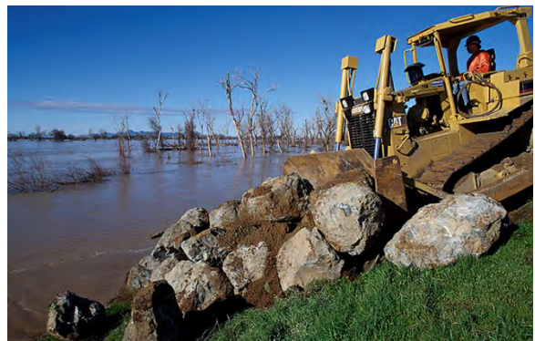
Many vulnerable Delta levees require installation of rock revetments, riprap, or other engineered structures along eroding banks to reduce erosion and protect levee foundations.
